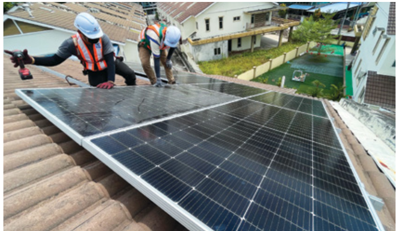
Figure 1: Installation of Solar Panel for NEM project
