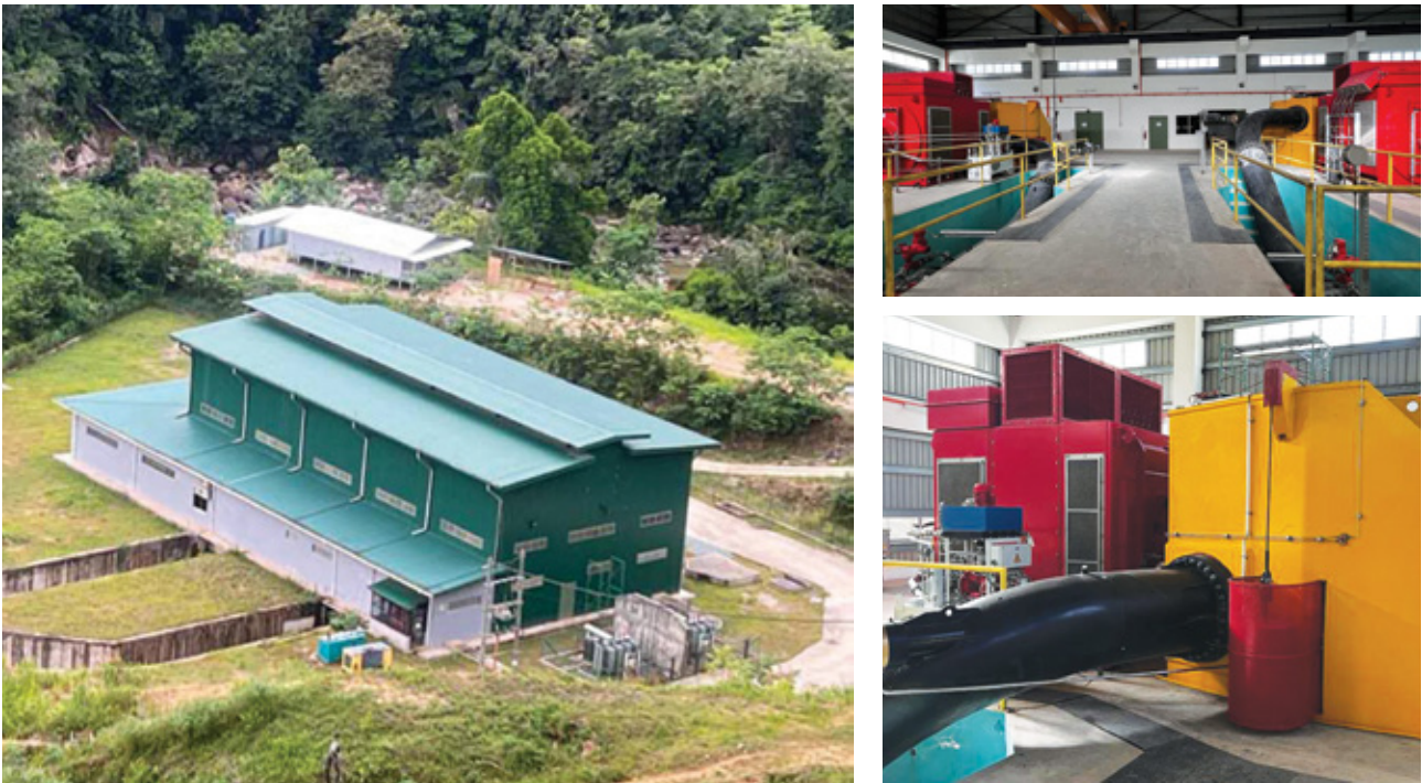
Figure 3 : Hydro Power Plant, Kota Marudu, Sabah
