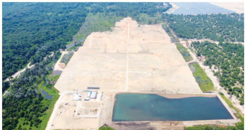
Figure 2 : Progress Photo at Pekan, Pahang
