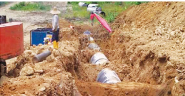
Figure 4 : Progress Photo at Kampar, Perak
